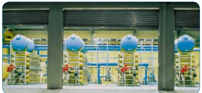
This Culligan Reverse Osmosis Desalination Plant churns out approximately 2.4 million gallons of water per day
